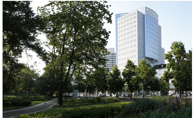
Quadoro headquarters in Offenbach, Germany
